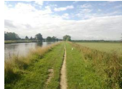
The canal corridor Picture by Ruth Greenwood
