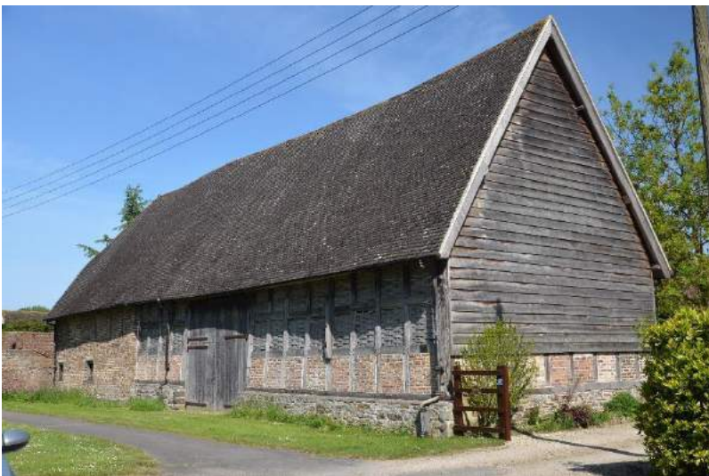
Grade 2* listed barn, part Frampton brick with square interwoven wattle panels. Photograph by Joy Greenwood
